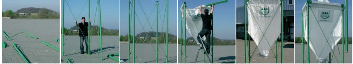
Example for an assembly of an animal feed silo
